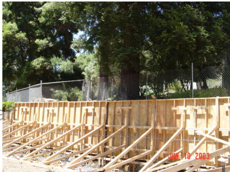
**A suggested minimum distance is 25 to 30 feet from excavation cut to tree trunks.**
