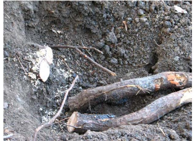
Woody roots shall not be shattered or broken in any way as a result of site activities. Shattered or broken areas shall be hand dug back into clear healthy root tissue and re-severed at right angles to root growth direction under the direct supervision of the project arborist (PA). Immediately (same day) backfill over roots and heavily irrigate (same day) after backfill to saturate the uppermost 24 inches of the soil profile.
