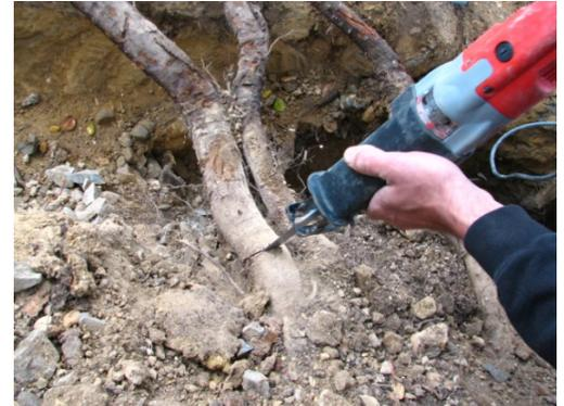
growth using sharp hand tools such as professional grade loppers, hand shears, chain saw, A/C sawzall, or other tools only under his/her direct supervision. See spec images at right. Note that a Sawzall blade indicating use for "bimetal" or "demolition" is typically not a good choice for this work. Instead, opt for a relatively large-toothed blade that indicates use for "pruning" or "wood" (see images at right).
