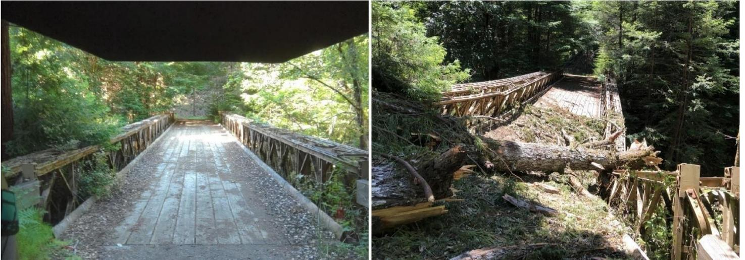
*Figure 7 Baker Fire Road Bridge before (left) and after (right) tree damage*
