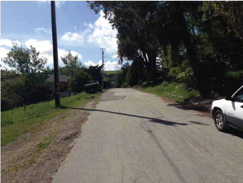
Photo 2: Node 048A Area Overview (West)
