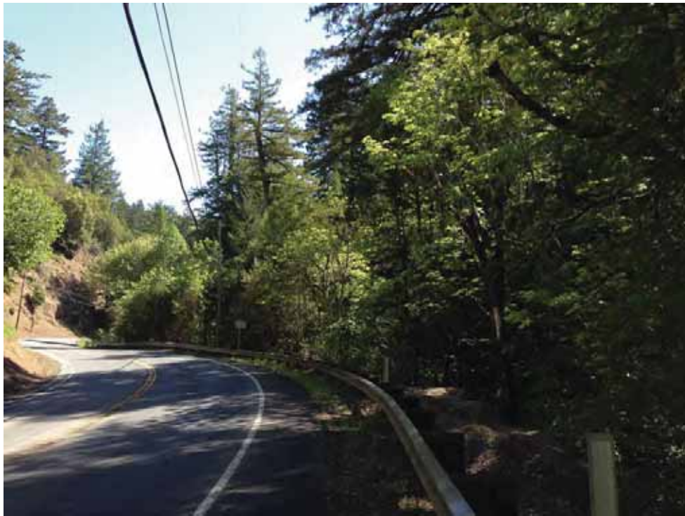
Photograph 3 View north of proposed Node 049A site.
