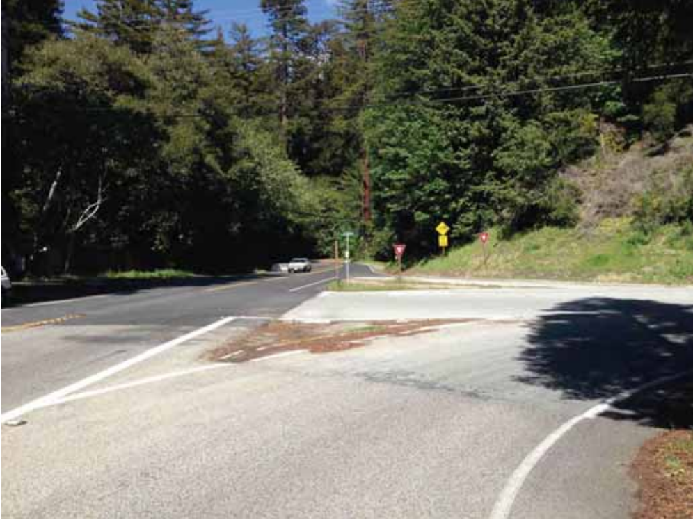
Photo 1: Node 047B Area Overview (North)
