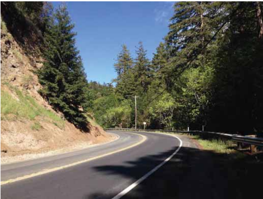
Photo 4: Node 049A Area Overview (East Northeast)
