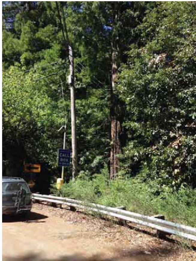
Photograph 4 View southwest of proposed Node 050A site.
