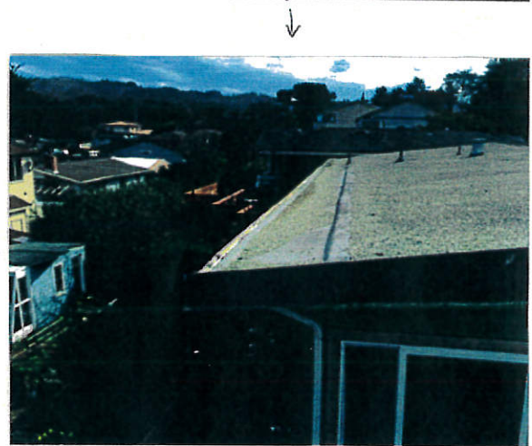
Photos taken from rooftop 315 Fifth Street towards the East
