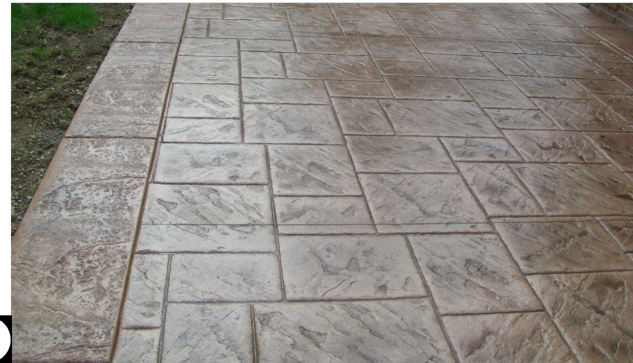
STAMPED CONCRETE AT DRIVEWAY ENTRANCES
