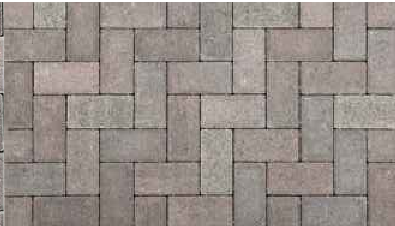
PERMEABLE PAVERS AT DRIVEWAYS (HERRINGBONE PATTERN)
