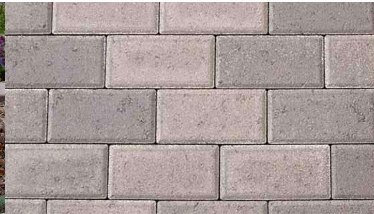
PERMEABLE PAVERS AT DRIVEWAYS (RUNNING BOND)
