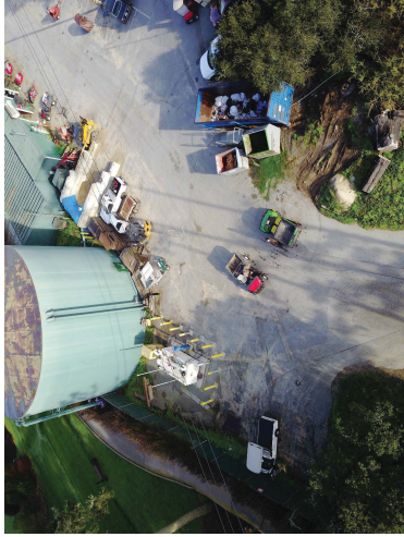
6 FUEL TANK AREA
