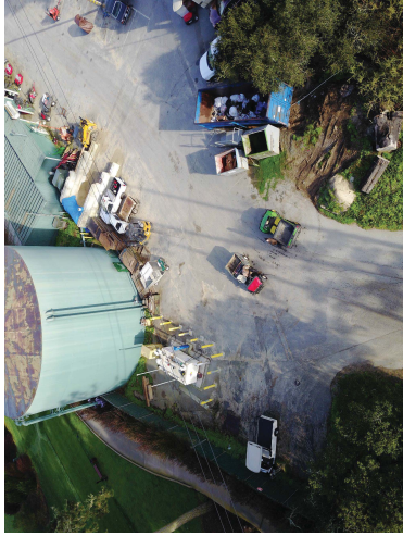
6 FUEL TANK AREA
