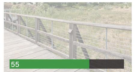
Example of a wooden guardrail with cable wire fencing
