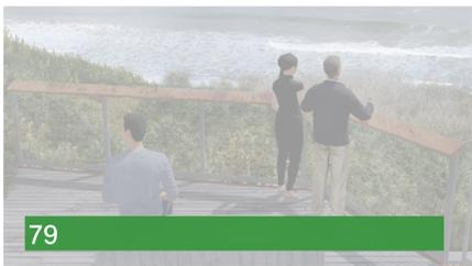
Guardrail with metal posts, wire cables, and a wood cap
